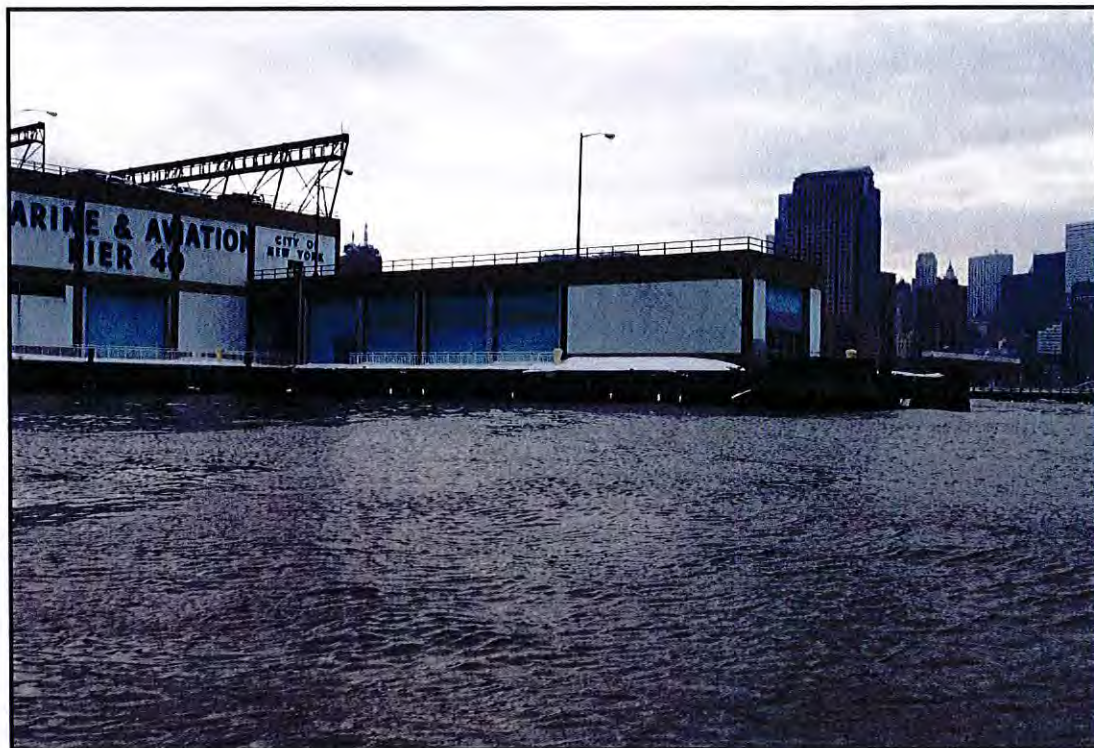
Photo B-2: Overall view of the Finger Pier Extension with one-story shed, looking southeast.
