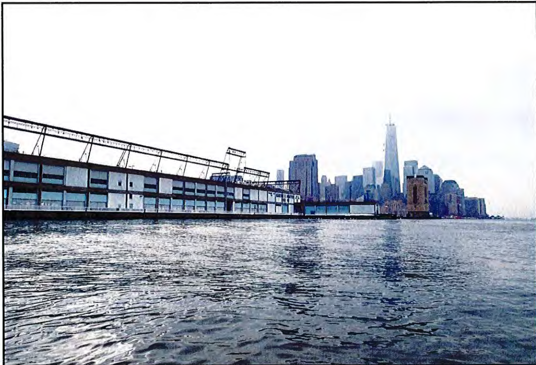
Photo B-1: Overall view of Pier 40, looking southeast.
