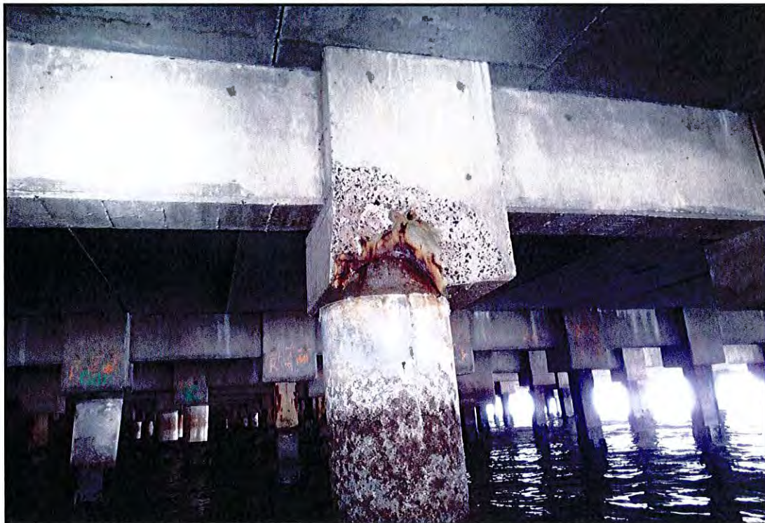
Photo B-10: Close-up of typical concrete encasement at the top of a steel H-pile at Bent S Pile Row 4.7.
