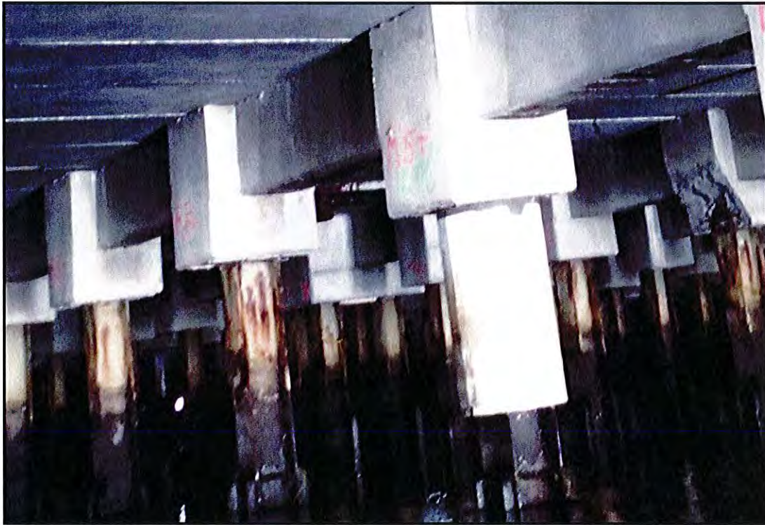
Photo B-9: Typical concrete encasement at the top of a steel H-pile in Bent F-bar (foreground) and typical epoxy coating at top of steel H-pile in Bent F-bar (background).
