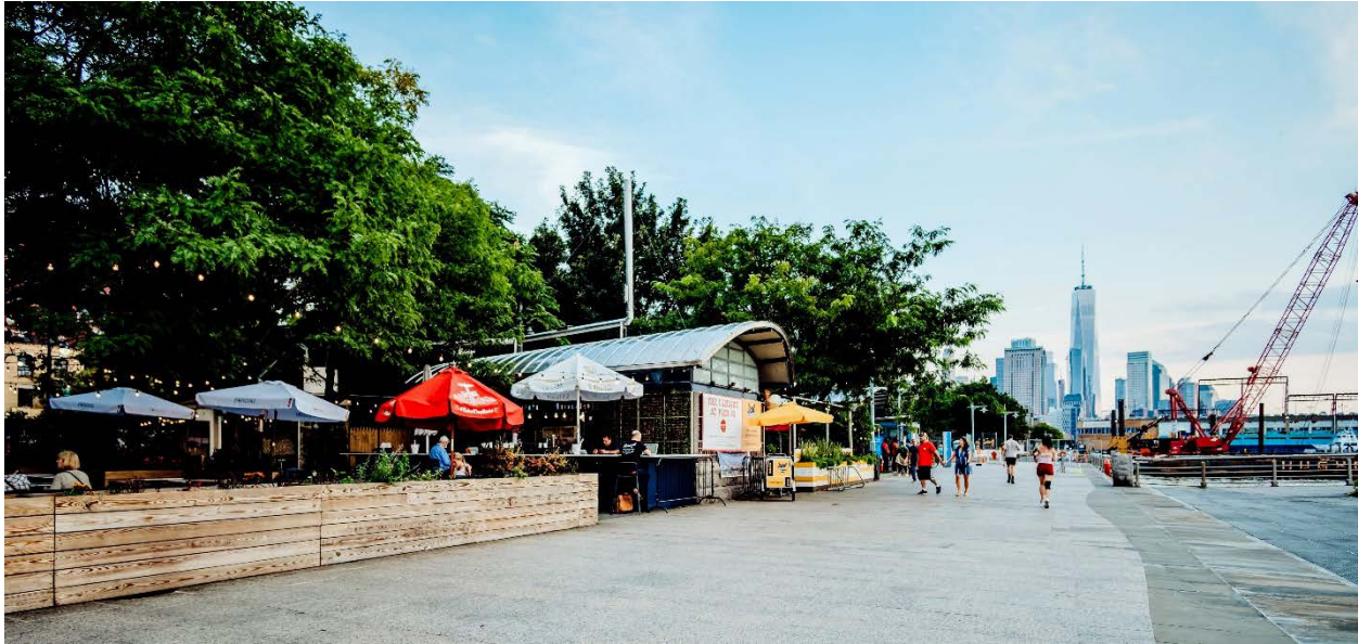
View of the Pier 45 Building and outdoor Seating Areas looking south
