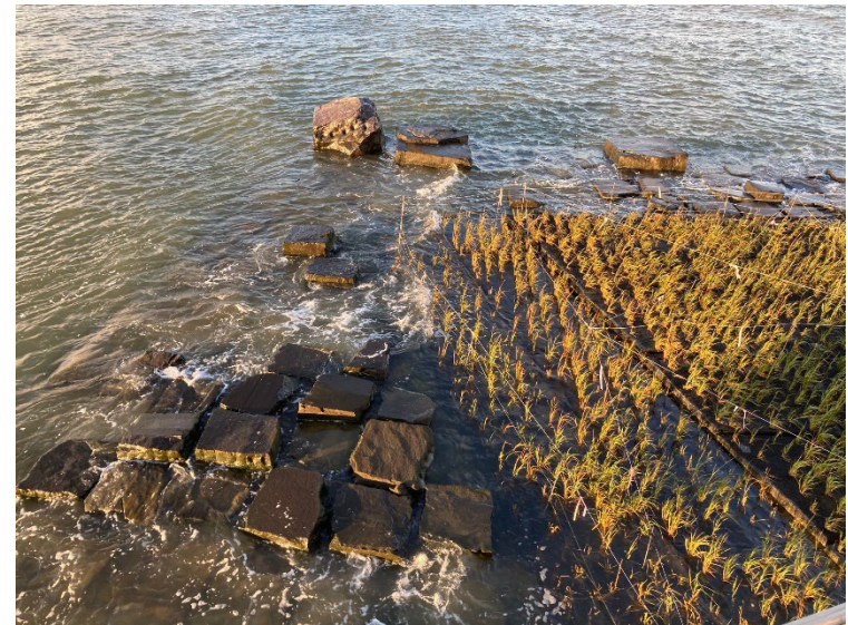
Fig. 2 | Northwest corner of Pier 26 tide deck, 3.5 hours after low tide
