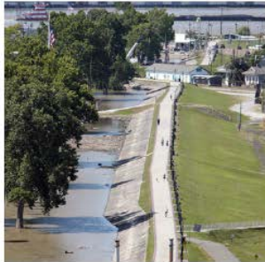
Levees: Embankments located at the shoreline that provide protection from flooding.
