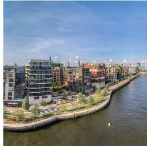
Elevation of Land and Streets: Elevation of existing or new development sites and streets above the expected storm level to protect from flooding.
