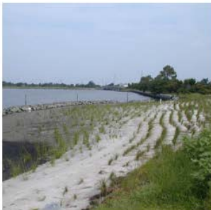
Living Shorelines: A bank stabilization technique that uses plants, sand/soil, and limited use of hard structure to provide shoreline protection and maintain valuable habitat.
