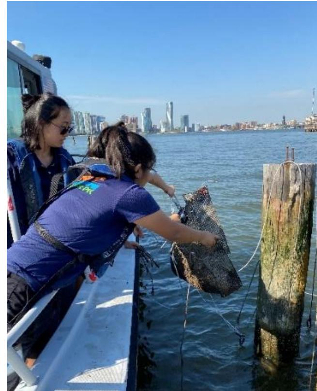
**Fig. 2** | Oyster wrap on a pile in deployment process.
