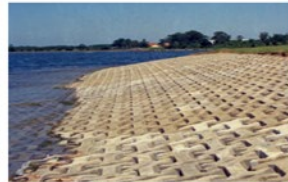
Revetments: Shoreline structures typically made of stone rubble or concrete blocks placed on a sloped surface to protect the underlying soil from erosion and reduce the force of wave action.
