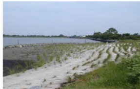
Living Shorelines: A bank stabilization technique that uses plants, sand/soil, and limited use of hard structure to provide shoreline protection and maintain valuable habitat.
