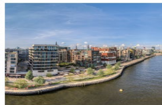
Elevation of Land and Streets: Elevation of existing or new development sites and streets above the expected storm level to protect from flooding.
