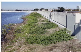
Floodwalls: Permanent or deployable walls used at the shoreline or upland to prevent flooding.
