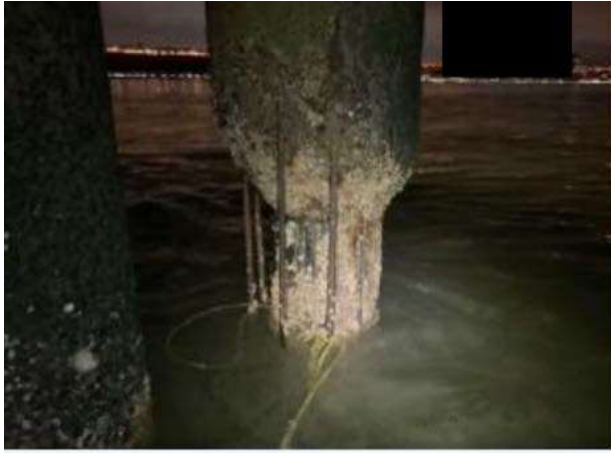
Spalled concrete
