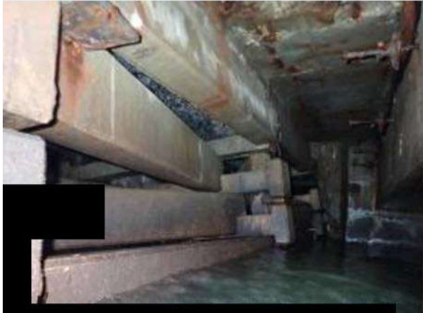
Marine borer damage
